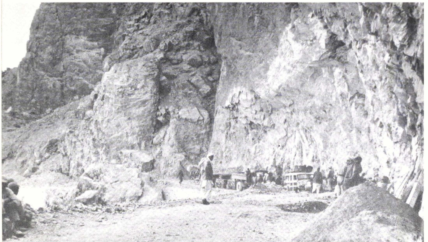
Blocked road to Jalalabad
